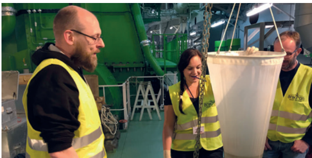
Ankron Water Services began testing a BWMS installation on a large container ship in May (Credit: Ankron Water Services)
